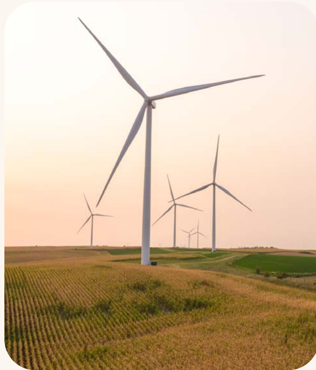
▲ Plum Creek wind farm (photograph provided by Ørsted A/S)
